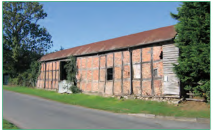
Large-scale timber-framed barns testify to the development of large arable-based farms across much of this area, often alongside and intermingled with a wide variety of farmstead types and scales. This example was converted into cattle housing and reroofed in corrugated iron in the early 20th century.
