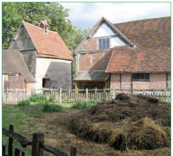
Fine farms, some ornamented with dovescotes as here at Mary Arden's House at Wilmscote, developed along the Avon Valley from the 15th century.
