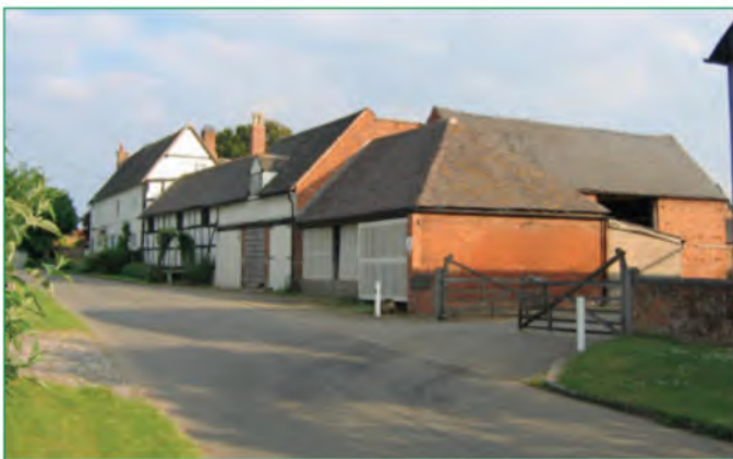
Large farmsteads also developed within and particularly on the edge of villages where they could more easily expand, as here in the Avon Valley. This group comprises a 17th century or earlier house, an attached stable or cowhouse and threshing barns, all in timber frame partly reclad in brick.
