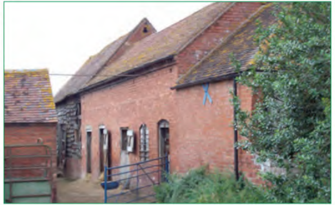
Mid 19th century brick stables with characteristic split-level doors.
