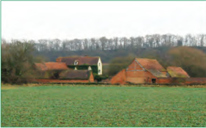
A defining characteristic of this area are the loose courtyard groups with working buildings to three or more sides of the yard. Those with timber-framed barns (typically of five bays) and other buildings (principally stabling and cattle housing) had developed into their present form by the 18th century. Buildings in brick and stone were later added, but these groupings are distinctive and significant for their early date where they survive.
