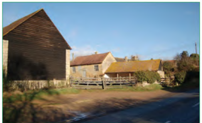
A loose courtyard group built of lias limestone in the south east of the area.
