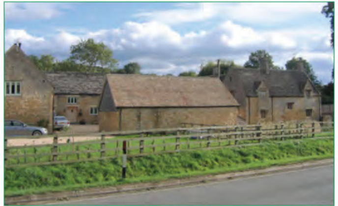
Many L-shaped groups developed into larger steadings with working buildings to additional sides of the yard: these are a distinctive characteristic of the arable vales across the south of the West Midlands. This group built in limestone, to the east of the area, relates to a 17th century house sited in land enclosed by this period.
