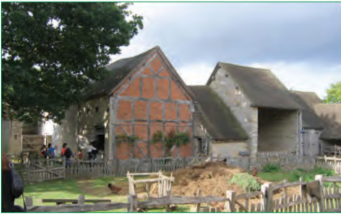
Other large farmsteads had developed by the 17th century into large complexes with two or more threshing barns, and a driftway providing access to the main yard. Evidence for early fabric is often concealed by later rebuilding in stone and brick: note the timber frame exposed in the gable end of the barn to the left of the driftway.
