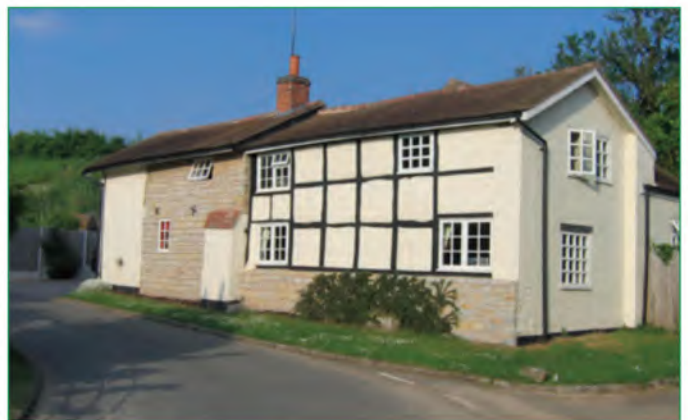
Linear farmsteads are hard to identify, and most had by the 20th century been converted to sole residential use.
