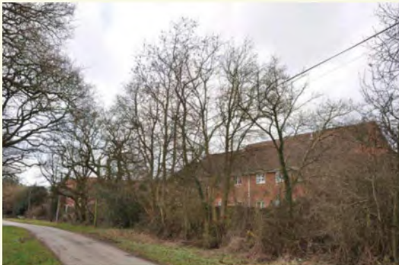
Viewpoint F4: Pumphouse Lane is overlooked by backs of houses on Great Hockings Lane
