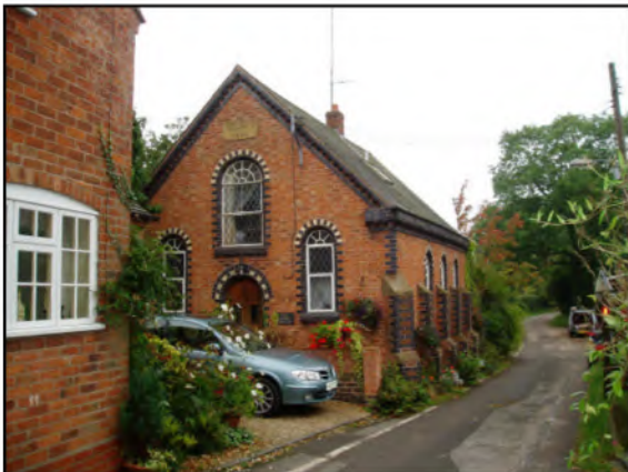
Fig 45: Former Methodist Chapel
