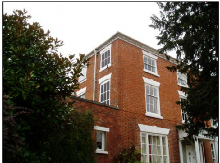
Fig 43: Blind windows painted to resemble glazing
