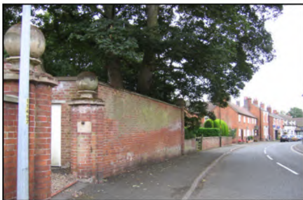
Fig 35: Street frontage with walled garden in High Street
