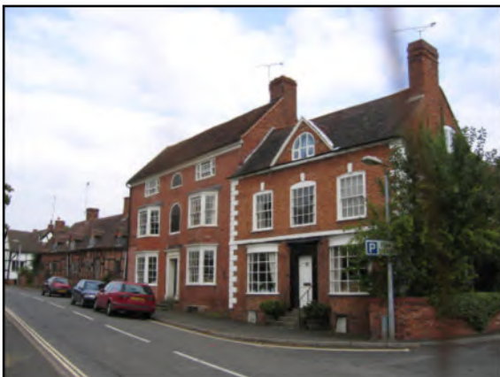
Fig 47: Buildings in High St
