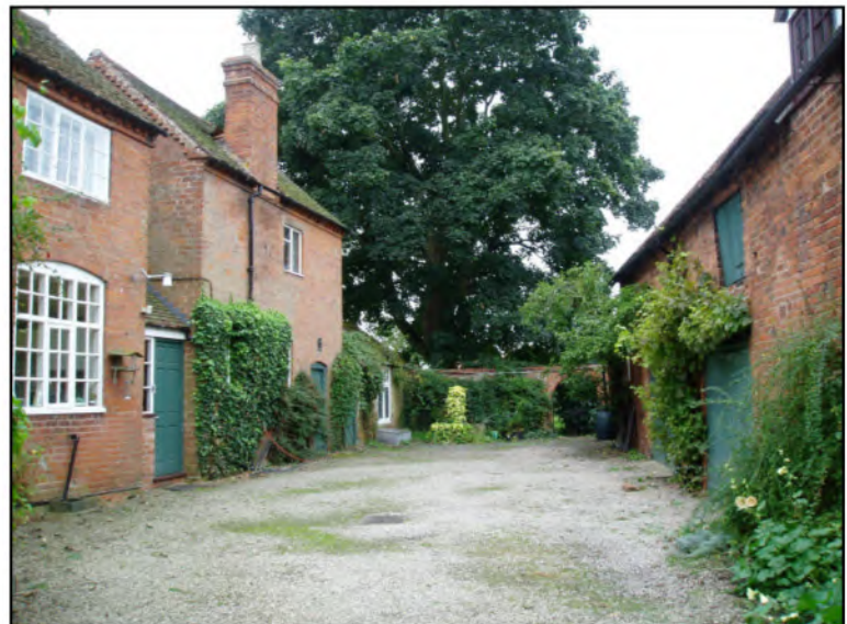
Fig 59: Yard adjacent No 41 High Street
