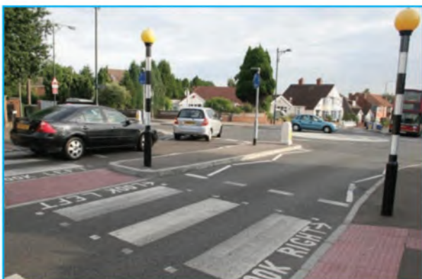
Zebra crossing close to mini-roundabout exit.
