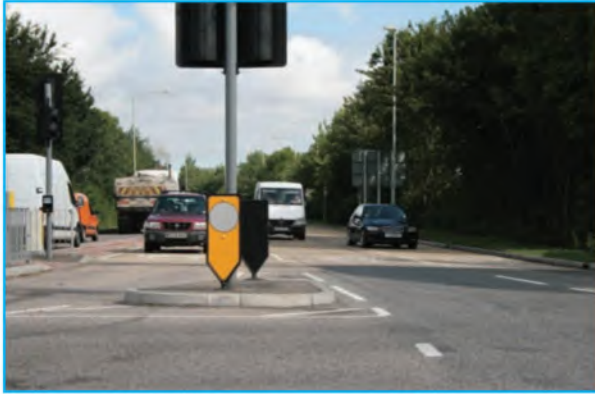
Keep left bollard, with rear face uncoloured
