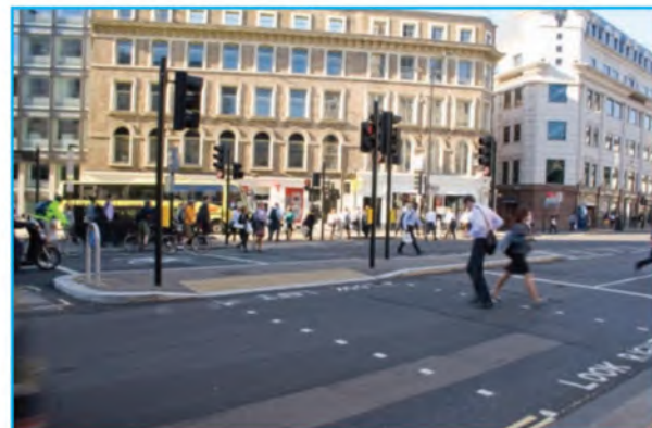
Staggered signalised crossing without guardrail
