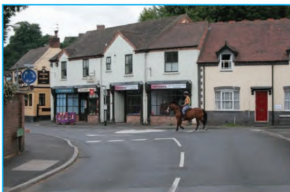
This mini-roundabout has an overall diameter of around 12m. It was installed as part of a village traffic calming scheme and has resulted in a significant reduction in collisions.
