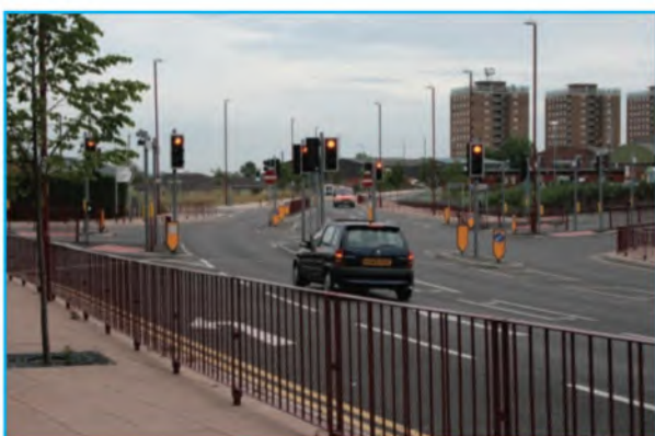
Newly-implemented highway scheme with extensive guardrailing
