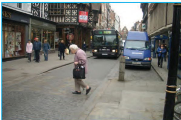
Shrewsbury High Street – ‘courtesy’ crossings are paved in the same material as the footways and line up with pedestrian routes on either side. See Traffic Advisory Leaflet 8/98 103 .
