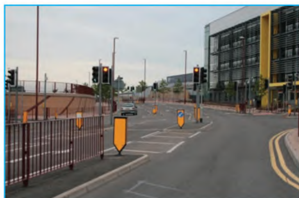
Multiple yellow retroreflective bollards can have a significant visual impact.
