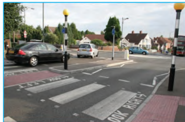
Zebra crossing located close to road junction.
