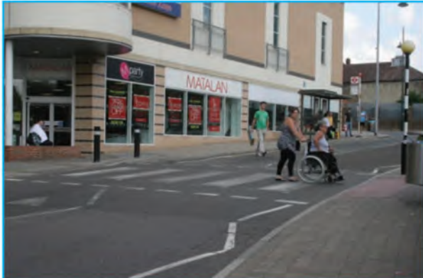
Zebra crossing on raised table.
