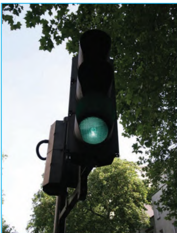
Signalised crossing with no white borders to signal heads
