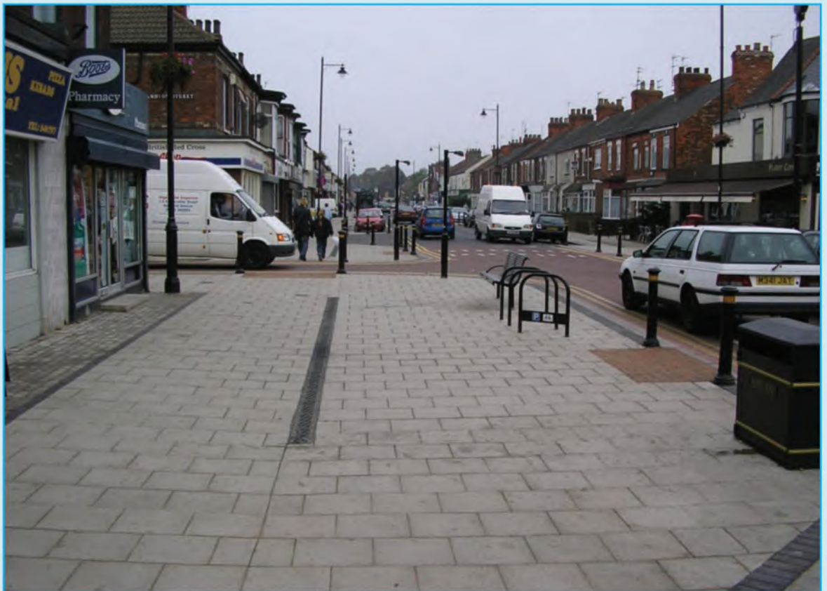
Footways widened significantly by narrowing carriageway
