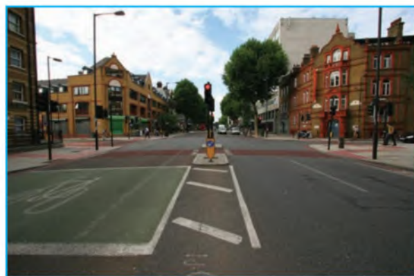
Traffic signal junction with clear and simple pedestrian crossings and advance cycle stop lines. Note lack of guardrailing and buildings close to junction corner, and tight corner radii.
