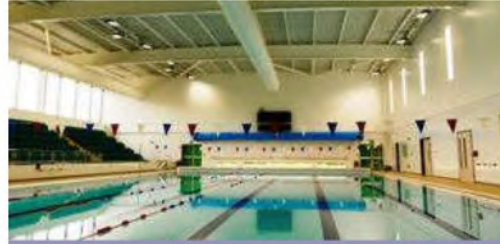
Abbey Stadium Sports Centre Pool
