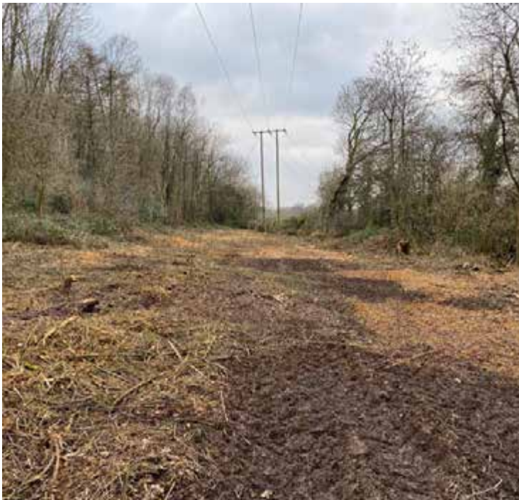
Image 3 Clearing beneath the power line
