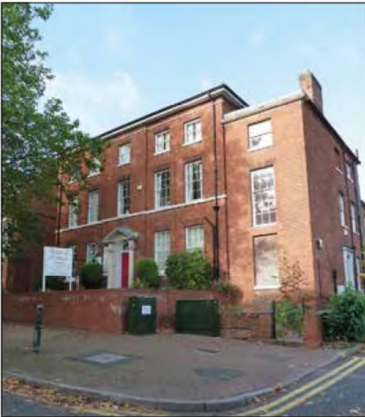
Red House, Church Green West
