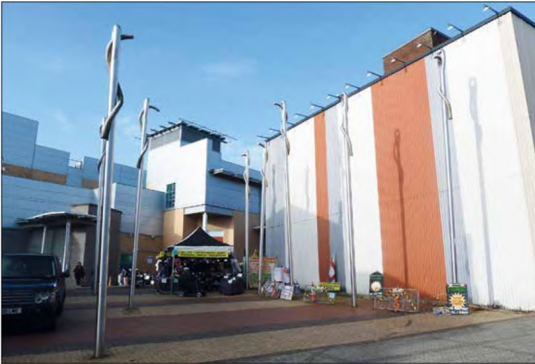
Part of the Kingfisher Centre to the south of the Conservation Area
