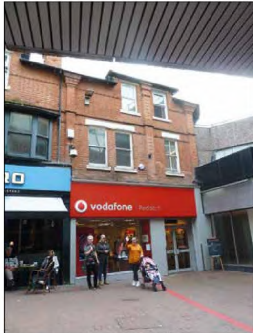
The oversized fascia to the Vodafone Shop in Evesham Walk
