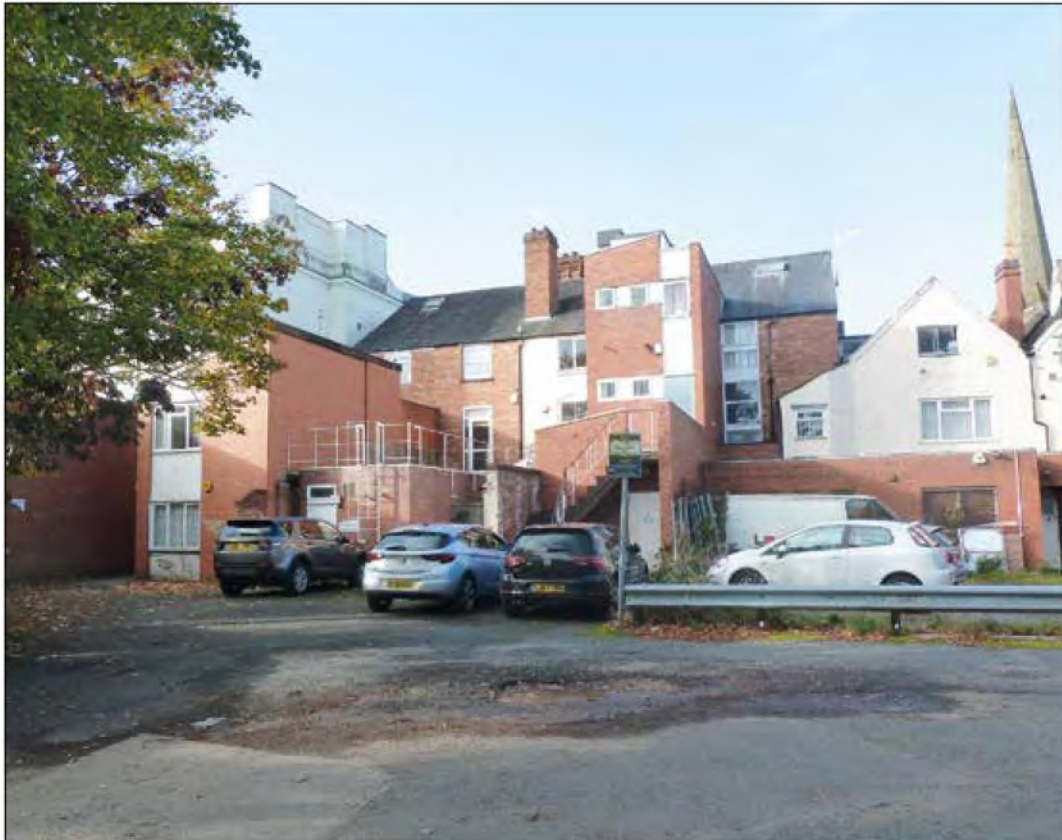
Poor rear extensions to properties on Church Green East
